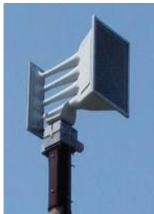
FCEM&HS continued work on narrowbanding of radios used in the Outdoor Warning Siren System. The project is due for completion by 2013. Story on page 4.
